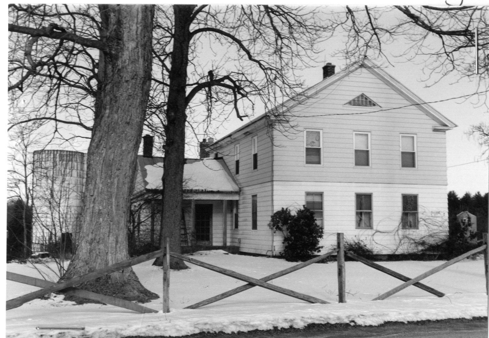
Phineas Strong House - 7 Moose Brook Road Looking north. Jan. 1998.
