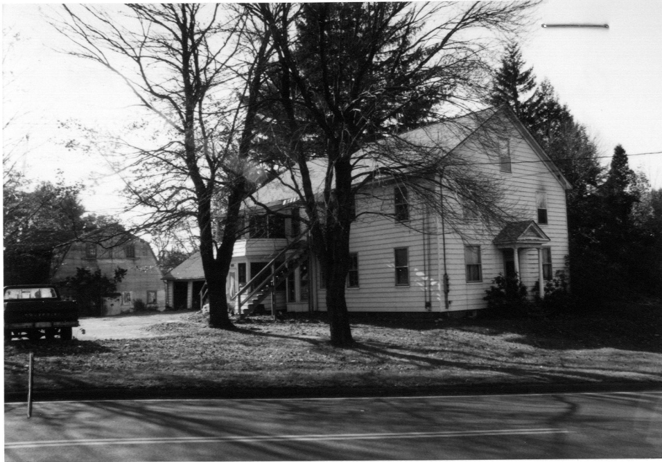
Canal storehouse - 100 Brickyard Road Looking northwest. Oct. 1997.
