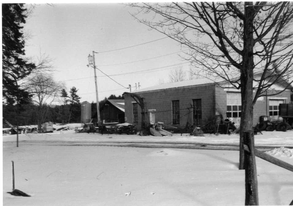
Phineas Strong House-outbuildings. 7 Moose Brook Road. Looking northwest. Jan. 1998.
