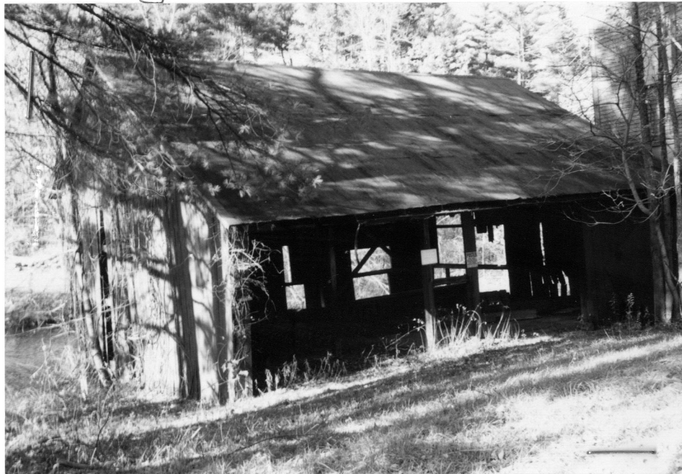
Lyman Mill, west end - at Manhan River east of Rt. 10, looking northwest. Oct. 1997.
