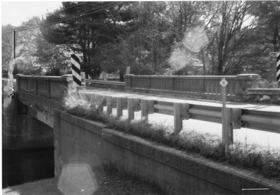
Bridge - College Hwy (Rt. 10) over the Manhan River. Looking SW. Oct. 1997.
