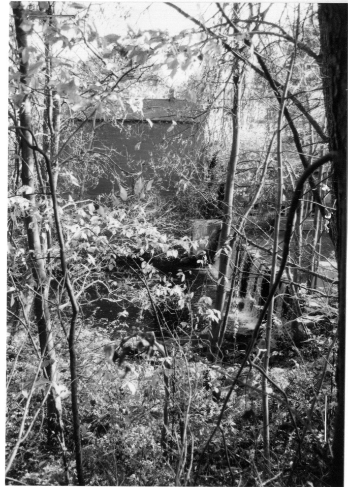
Lyman dam, mill in background, looking south. Manhan River east of Rt. 10. Oct. 1997.
