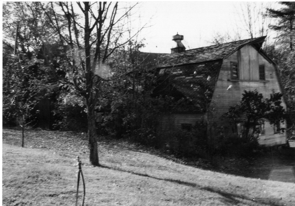
Canal storehouse barn - 100 Brickyard Rd. Looking northwest. Oct. 1997.
