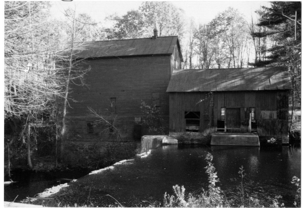
Lyman Mill and Dam at Manhan River, east of Route 10. Looking South. Oct. 1997.
