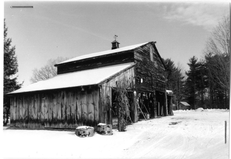
Harry Gorton House - 275 College Hwy. Looking southeast. Jan. 1998.
