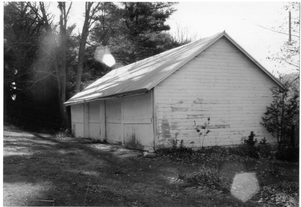
Canal storehouse - garage - 100 Brickyard Rd. Looking northwest. Oct. 1997.
