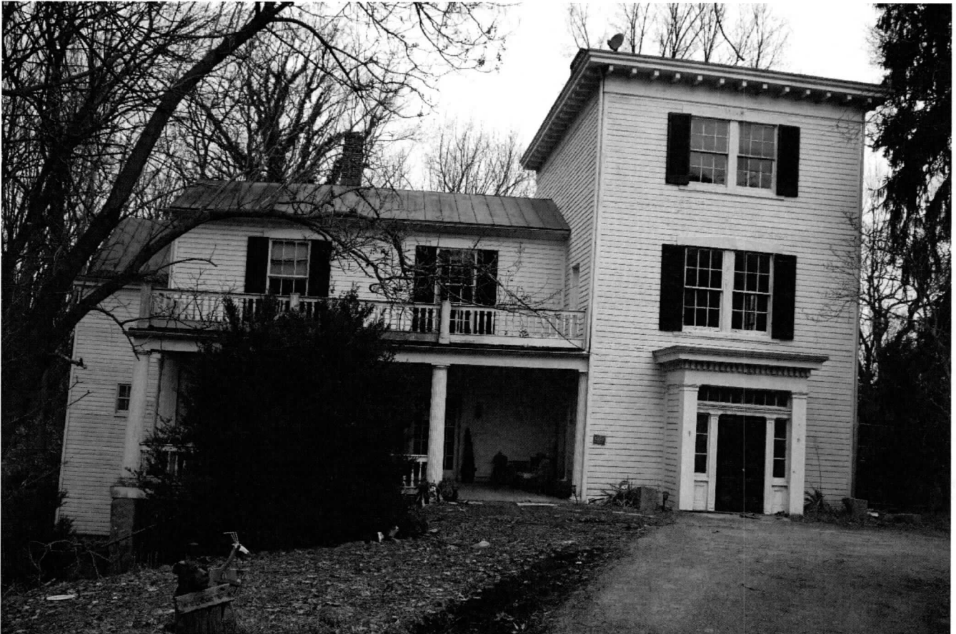
Photo 1 of 22: South elevation. 3/8/2019
