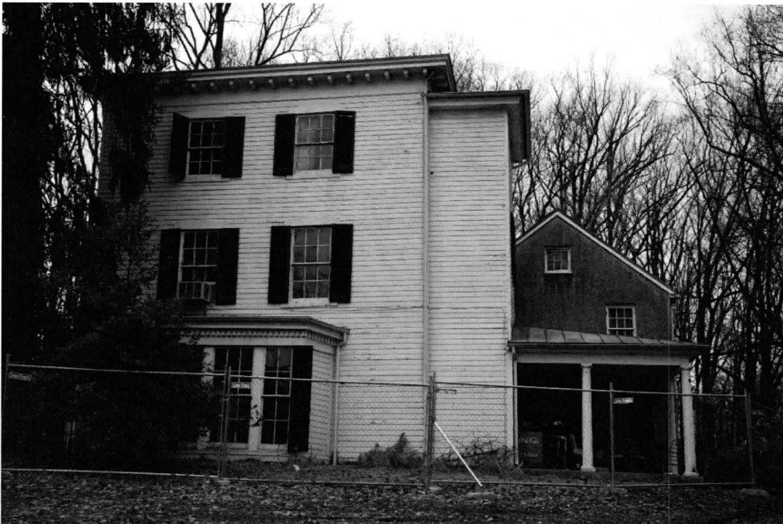
Photo 3 of 22: East elevation. 3/8/2019
