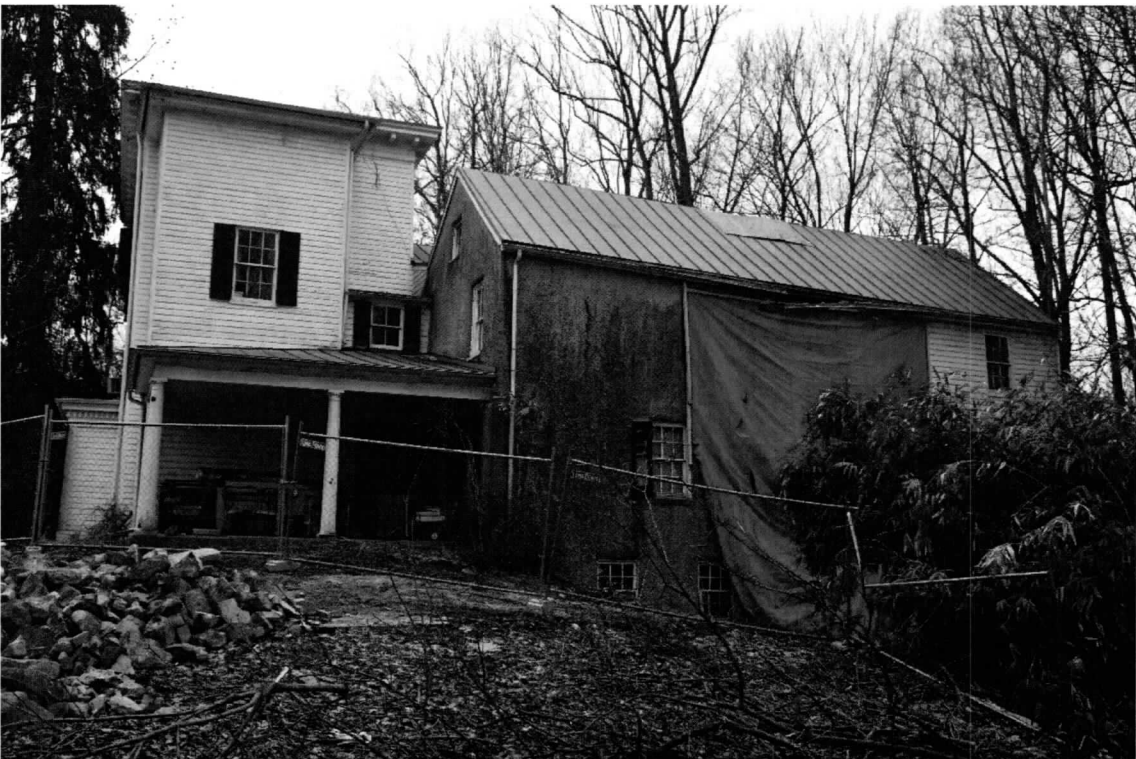
Photo 4 of 22: North elevation. 3/8/2019
