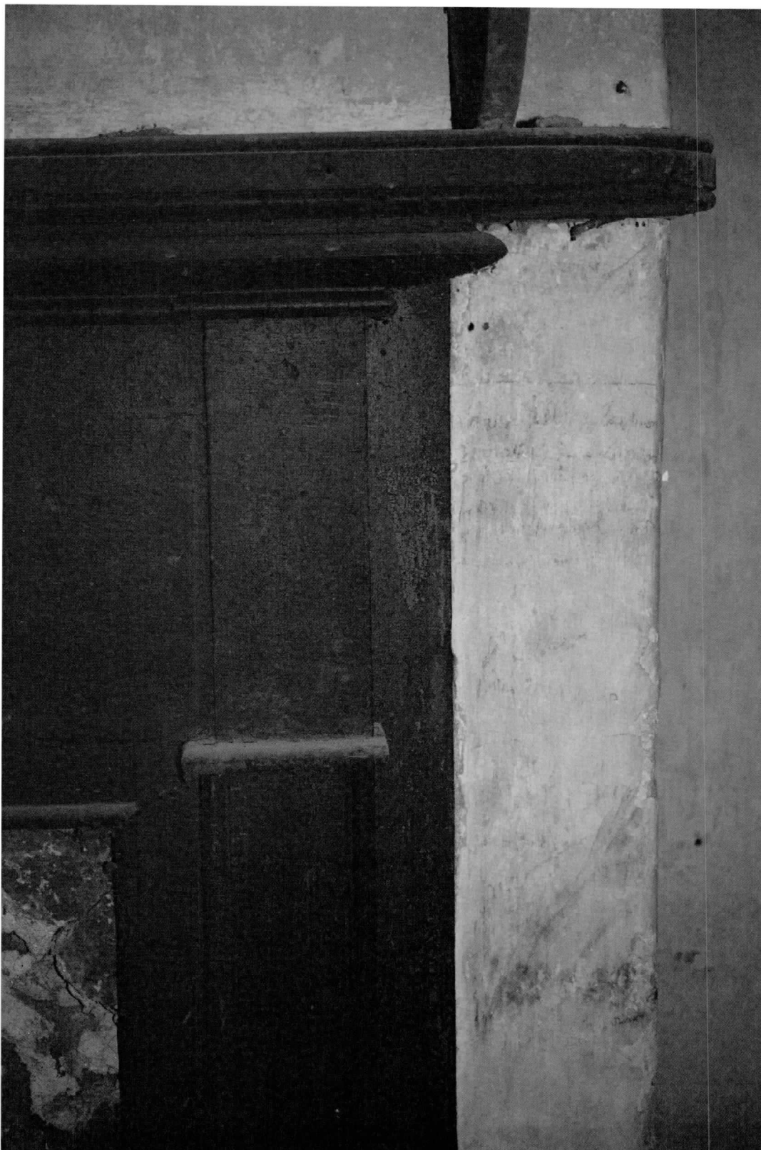
Photo 20 of 22: Basement, southwest room, mantel detail. 3/26/2019
