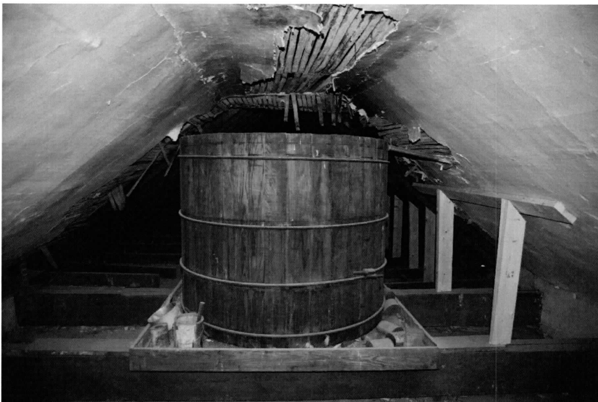
Photo 18 of 22: Cistern in attic of stone section. 3/8/2019
