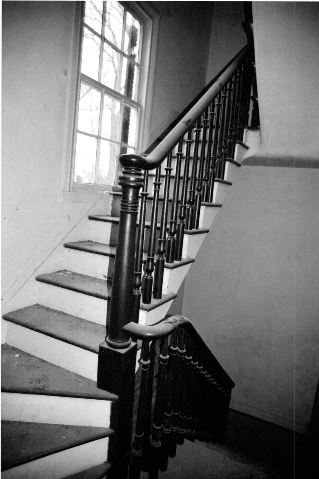
Photo 13 of 22: Second story stair passage, view northeast. 3/8/2019
