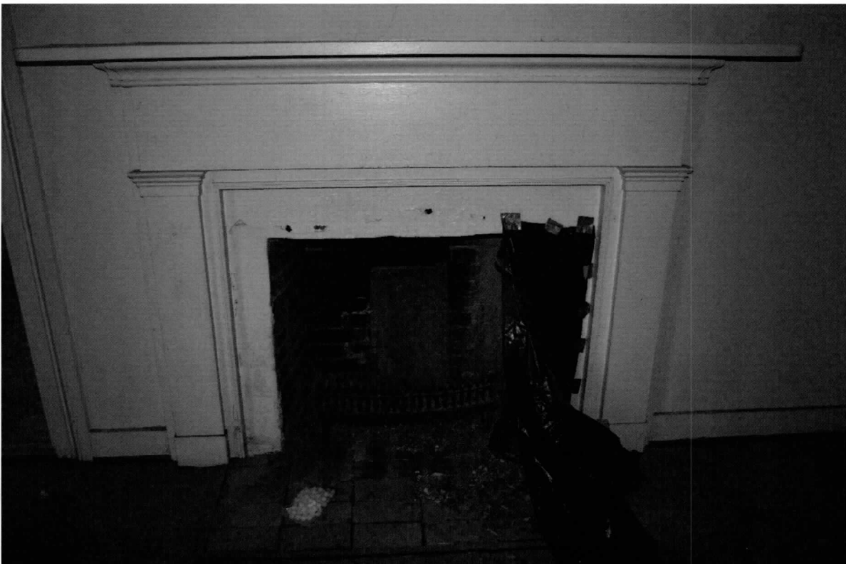
Photo 15 of 22: Second-story south-center chamber, mantel. 3/15/2019
