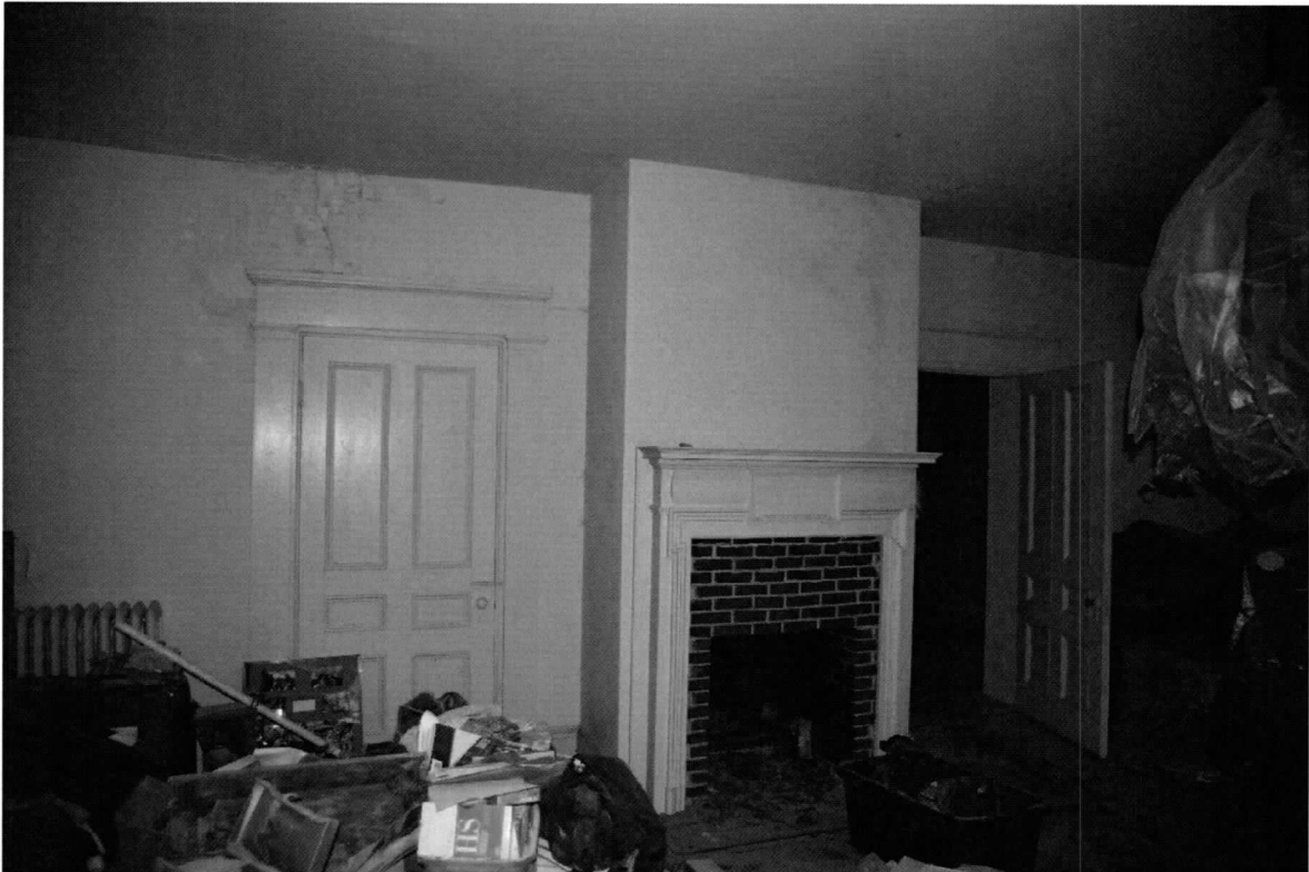
Photo 7 of 22: Southeast room, view northwest. 3/8/2019
