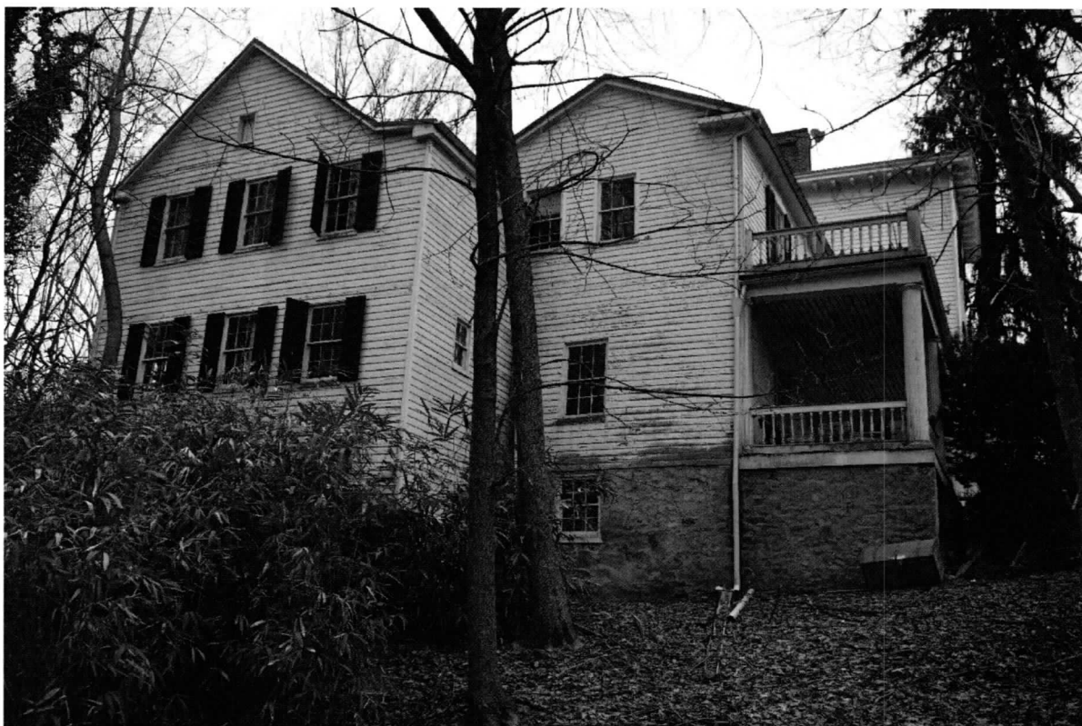
Photo 5 of 22: West elevation. 3/8/2019
