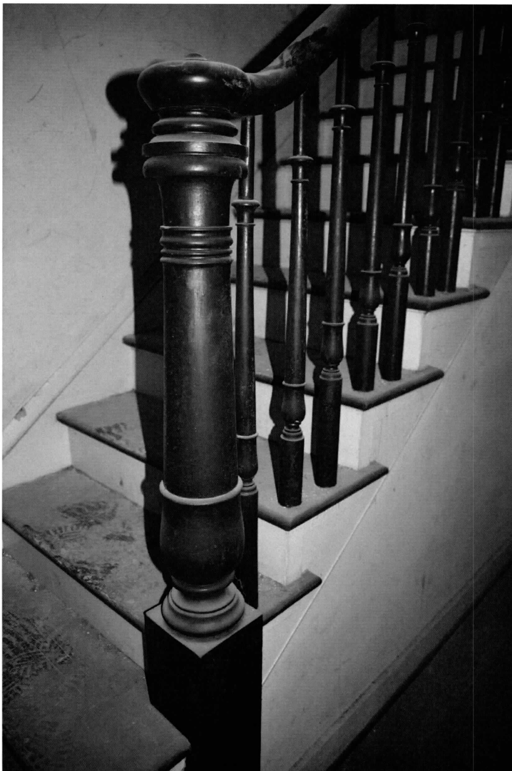
Photo 12 of 22: First story stair passage, newel. 3/8/2019
