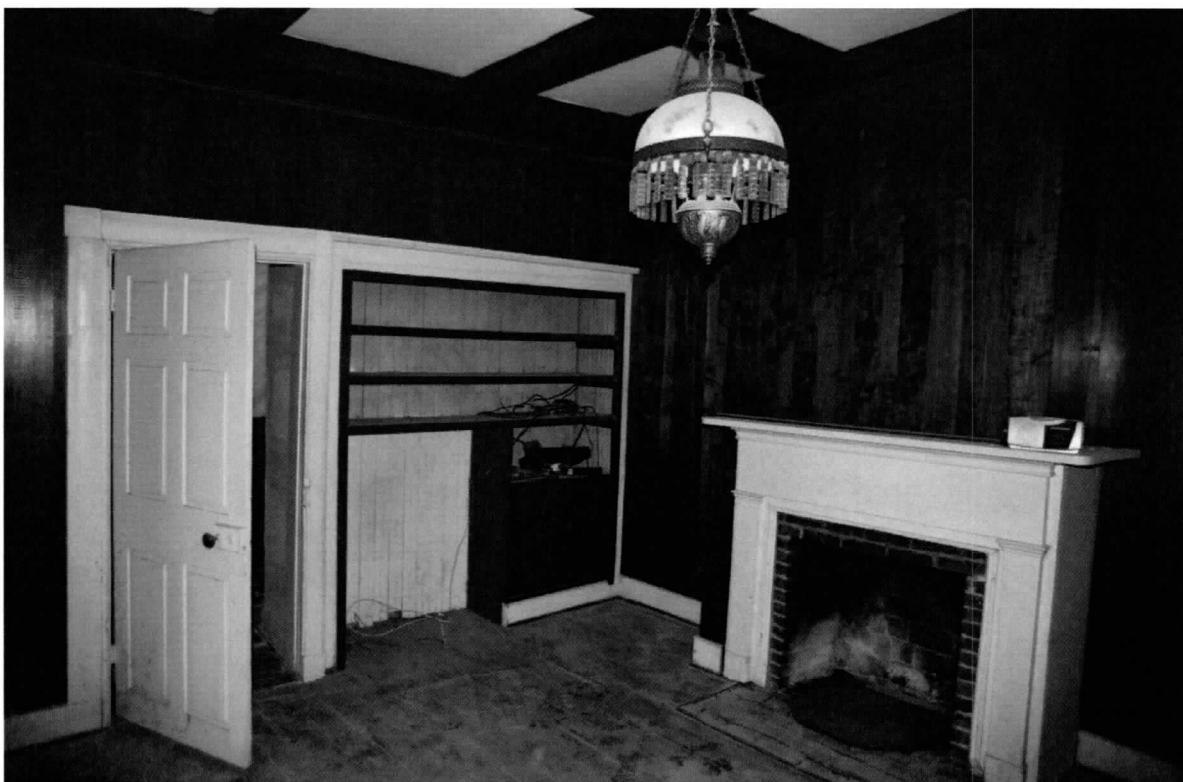
Photo 10 of 22: Southwest room, view northeast. 3/8/2019
