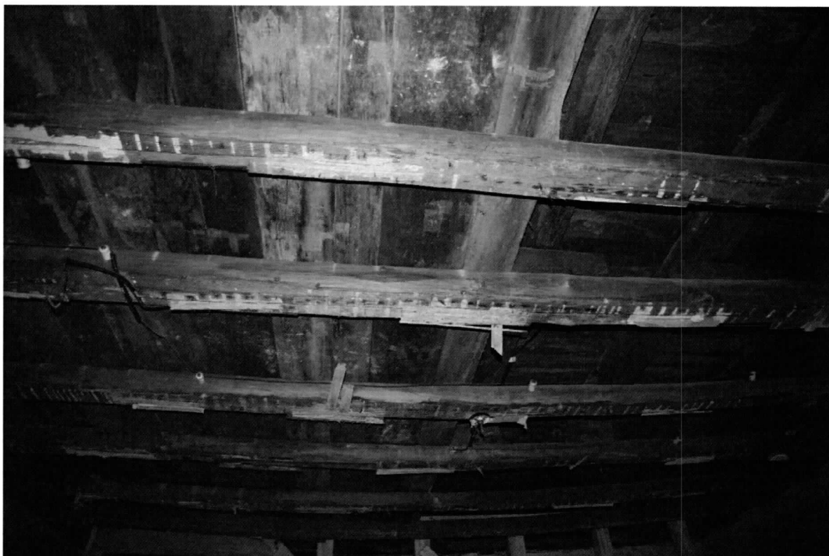
Photo 9 of 22: South-center room ceiling framing, view north. 5/9/2019
